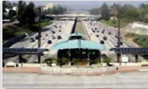
Recently completed solar photovoltaic canopies atop a Pasadena light rail station – a project that CEERT worked on for six years
