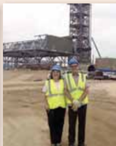
Katie McCormack of the Energy Foundation and CEERT Executive Director John White at the construction site of BrightSource Energy's Ivanpah solar thermal project
