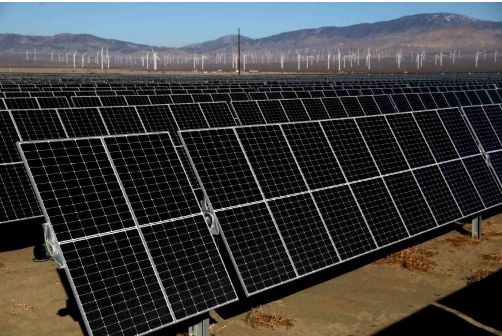
Solar panels track the morning sun at Rosamond Central, a newly completed 192-megawatt solar farm developed by Clearway Energy Group in California's Kern County, on Feb. 4, 2021, with wind turbines in the background. (Gary Coronado / Los Angeles Times)
