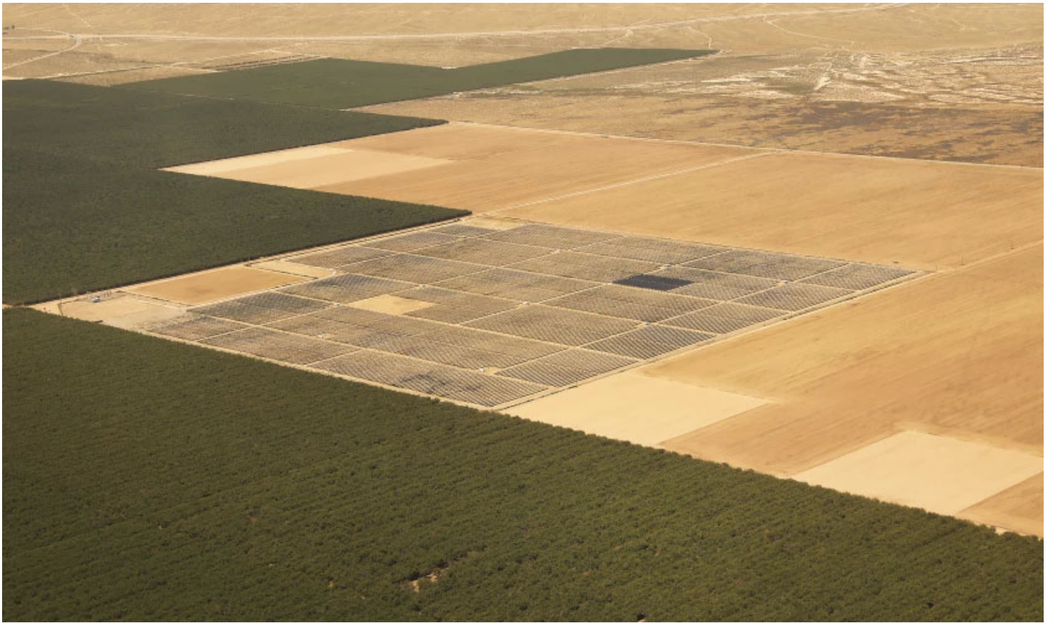
The 20-megawatt Maricopa West solar project, surrounded by almond groves, in California's Kern County. (Al Seib / Los Angeles Times)
