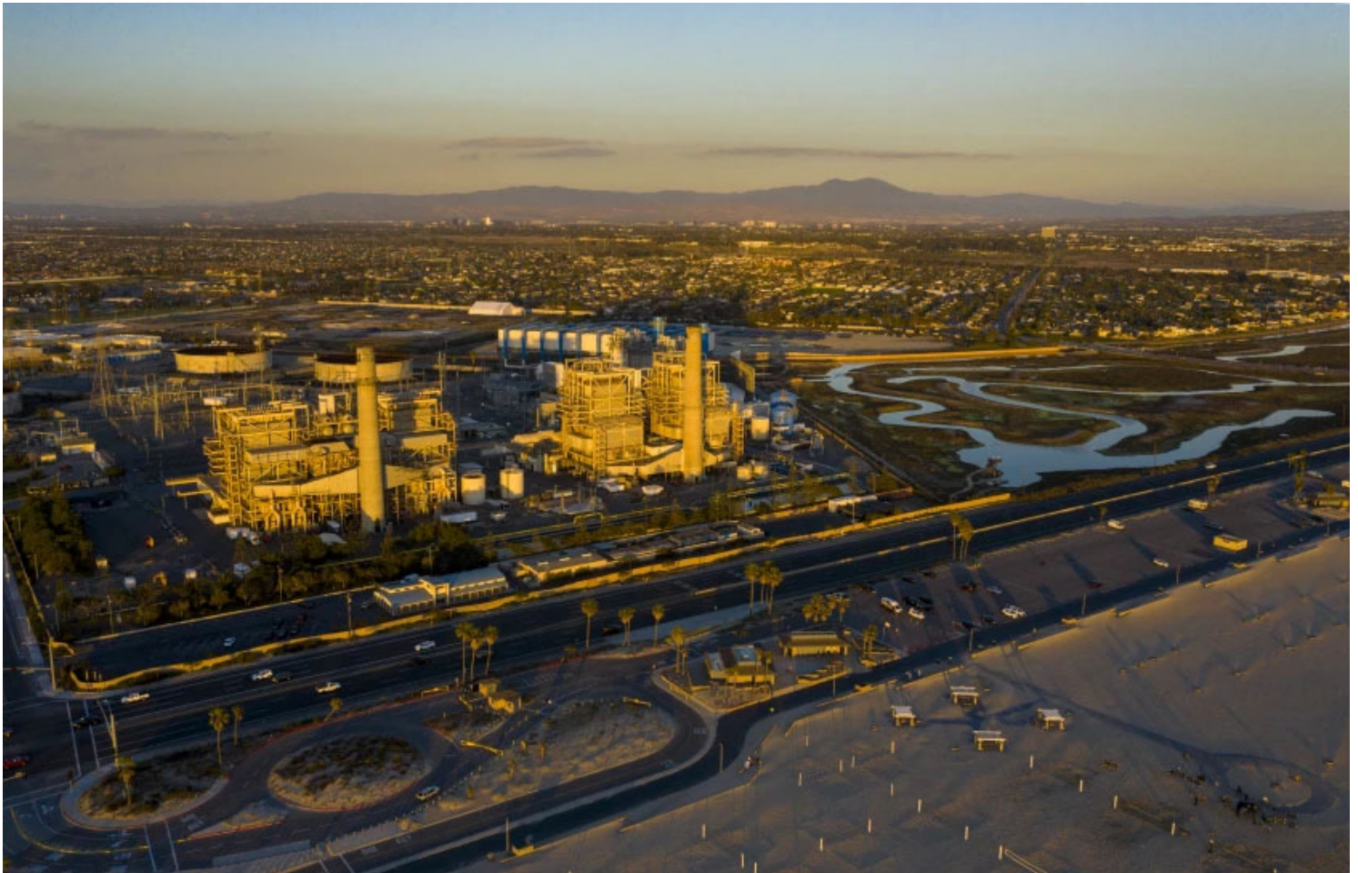
A gas-fired power plant owned by AES Corp. in Huntington Beach was the only one of the four coastal gas plants that was fully available during last month's heat wave. (Allen J. Schaben / Los Angeles Times)
