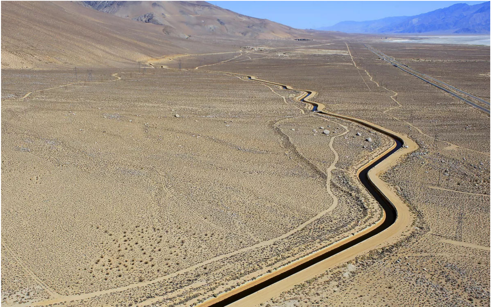
An aerial view of the Los Angeles Aqueduct as it flows south in its concrete-lined channel from the Owens Valley. (Brian van der Brug / Los Angeles Times)
