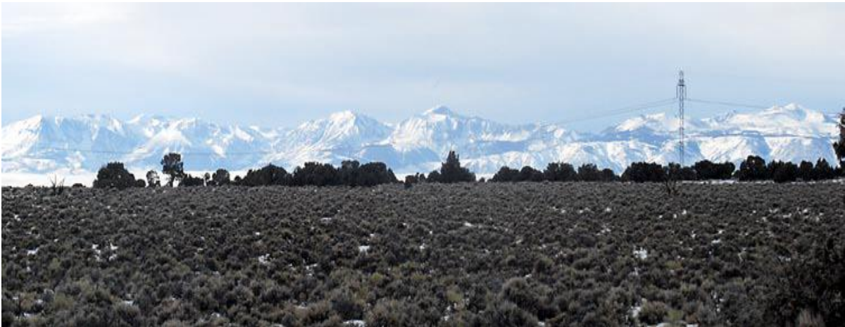
Pacific DC Intertie transmission line
