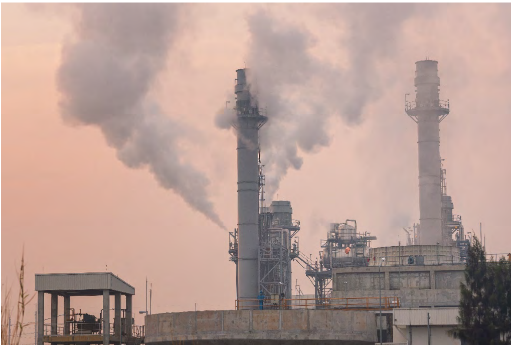
A gas-fired power plant
