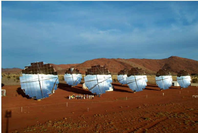
Figure A-8 Solar Systems Pty, Ltd: Parabolic Dish PV Concentrator (Source: NREL)
