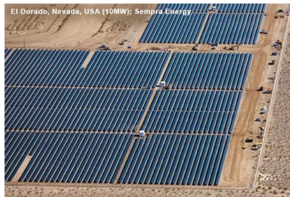
Figure A-7. 10 MW Large-Scale Thin Film Photovoltaic Power Plant, El Dorado, Nevada (Photo: Courtesy of First Solar)
