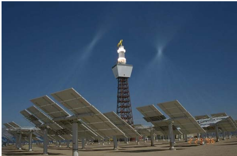
Figure A-4. 10 MW Solar Two Power Tower Plant, Daggett, California (Source: Sandia National Laboratories)
