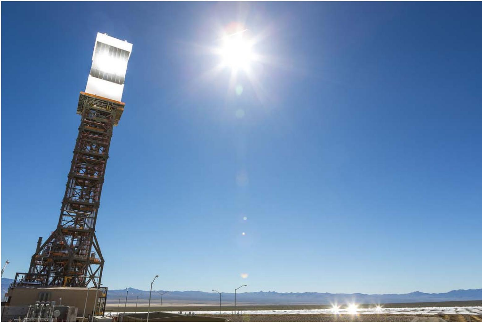
***The top of Tower 1 is "lit" during a steam blow test at the Ivanpah Solar Power Facility. Photo: BrightSource Energy***
