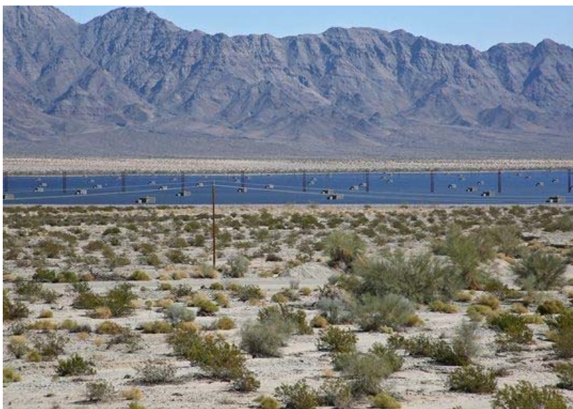
Open desert surrounds the Desert Sunlight solar project near Desert Center, in eastern Riverside County. At 550 megawatts, it's the world's largest solar power plant. (Photo: Jay Calderon/The Desert Sun)
