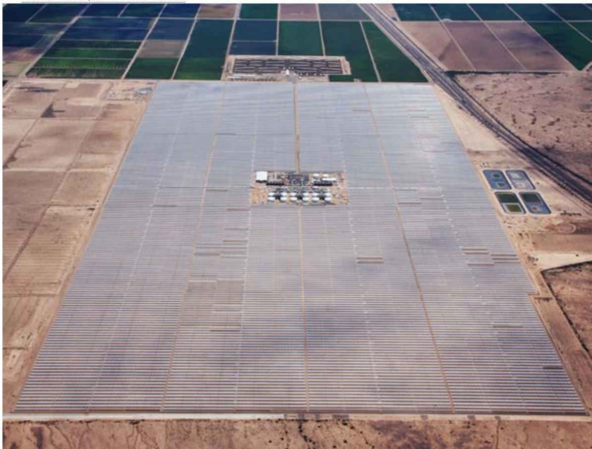
The Solana solar power plant near Gila Bend | Photo: Abengoa Solar
