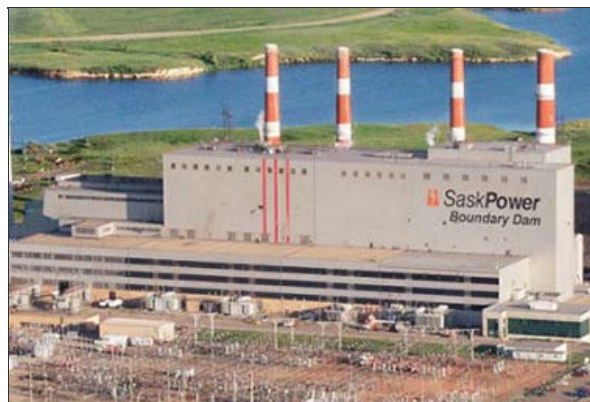
The Boundary Dam Power Station near Estevan, Saskatchewan, is one of more than 20 fossil fuel power plants worldwide that are being fitted with carbon capture and sequestration equipment as planners
