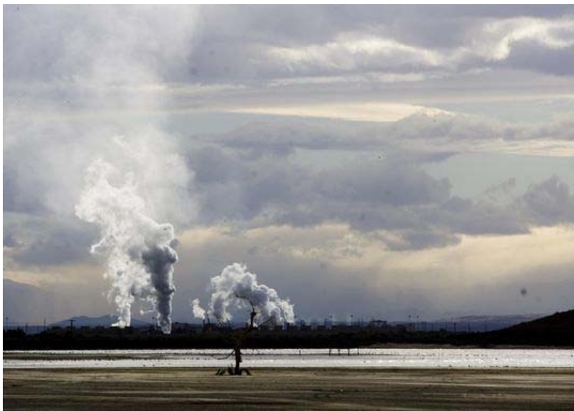
A geothermal power plant on the southern shore of the Salton Sea is visible from Red Hill Bay on Dec. 14, 2012. (Photo: Omar Ornelas/The Desert Sun)
