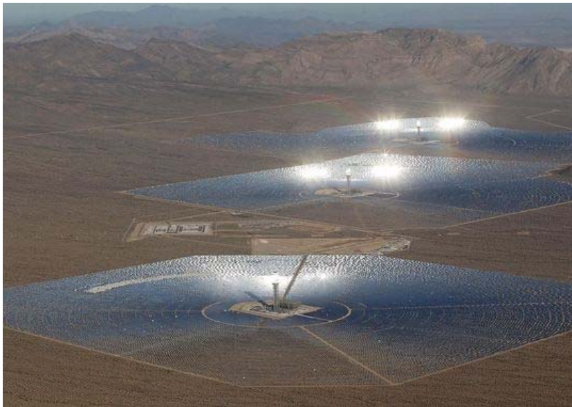
At the Ivanpah solar plant in San Bernardino County, mirrors focus sunlight on boilers at the top of solar power towers on Oct. 21, 2014. (Photo: Jay Calderon/The Desert Sun)
