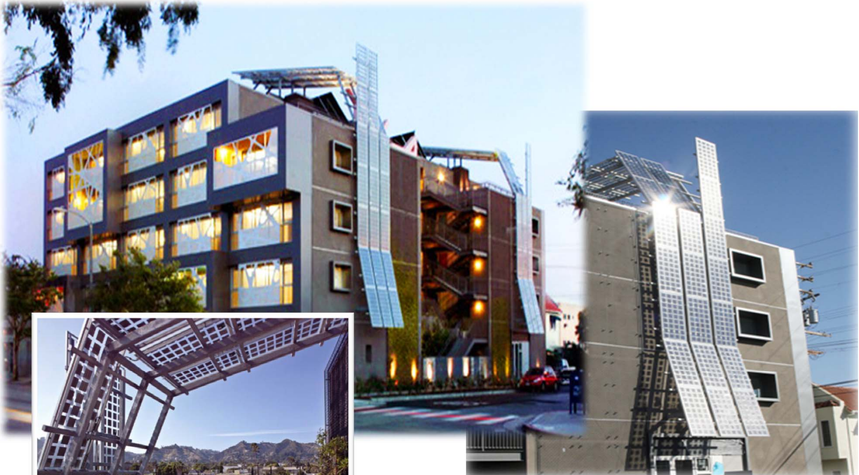
11kW Building-Integrated PV in Santa Monica, California. Energy powers common areas in the multi-use residential complex.
