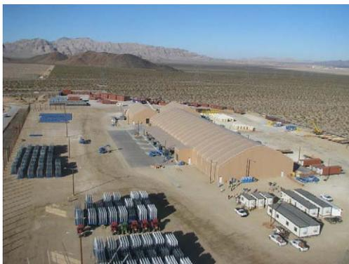
*The heliostat assembly building with mirrors ready for transport to the solar fie*
