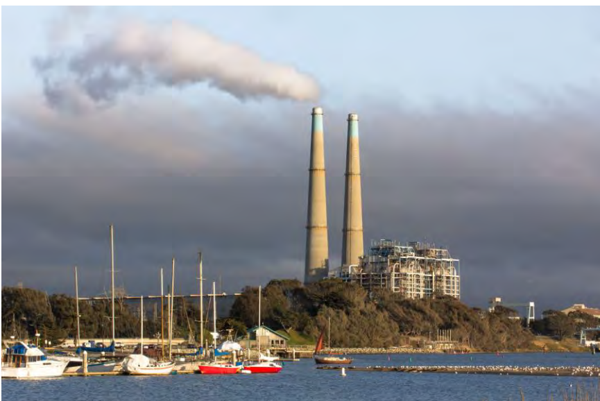
Moss Landing coastal gas-fired power plant
